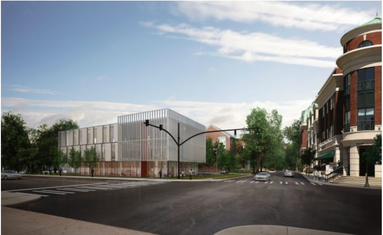
A view of the building from the corner of Main Street and Parkview Avenue.
